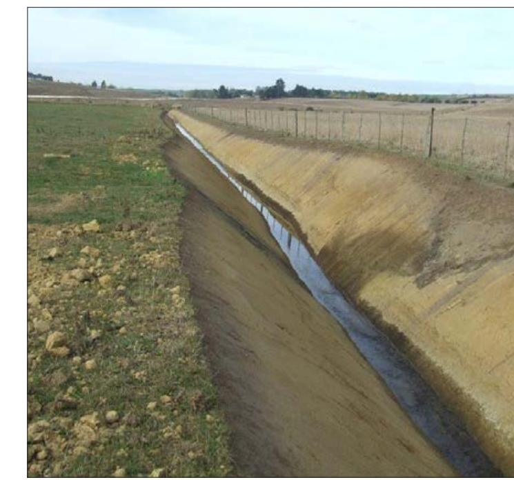
While this may look like a drain, it is a river that has been modified and straightened. (Friston Stream).
